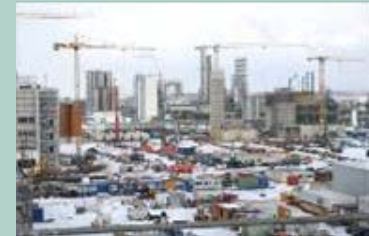
March 2010 View on construction site
