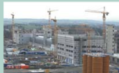
November 2009 Deposition reactor hall
