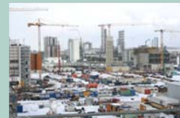
March 2010 View on construction site
