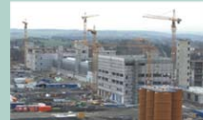
November 2009 Deposition reactor hall
