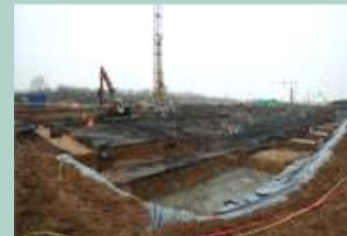
March 2009 Site preparation
