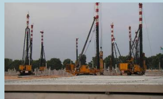
September 2006: Piling started
