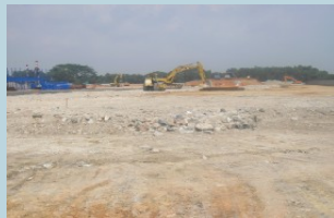
August 2006: Preparing the ground
