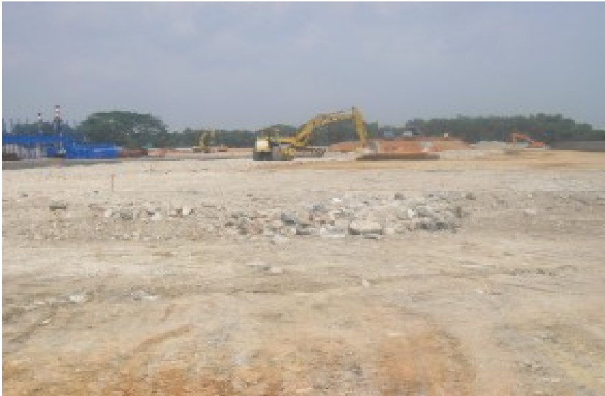
August 2006: Preparing the ground
