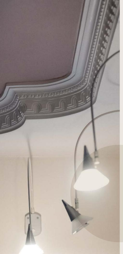
Plaster structures on ceilings are a typical and much sought-after feature of old buildings from the Wilhelminian era and can be replicated with silicone moldmaking compounds.
